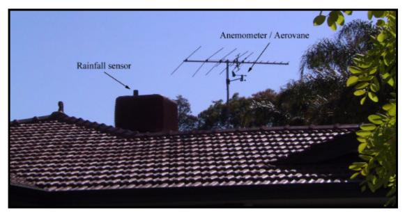
Figure 3.7 – On-site sensor placement.
